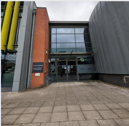
The front doors of Moore Building
