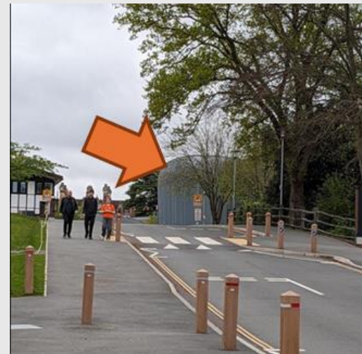
The Moore building from this angle.
